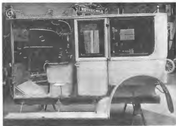
AN EXCELLENT EXAMPLE OF THE USE OF ALUMINUM FOR BODIES.
